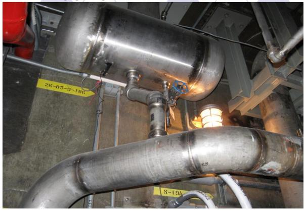
Developed at Diablo Canyon, a large tank is suspended above the high point of the pipe. This system will have seismic concerns, be expensive in implement and requires header space that may not be available in many cases. The system presents no way to measure the voids and must still use a vent to remove the voids.
