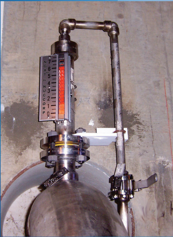
A typical NGAT-150 installation eliminates the need for ultrasonic testing. The goose-neck option allows for easy access to vent valve.
